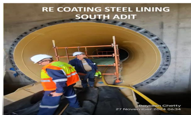
Figure 18: Re Coating Steel Lining
