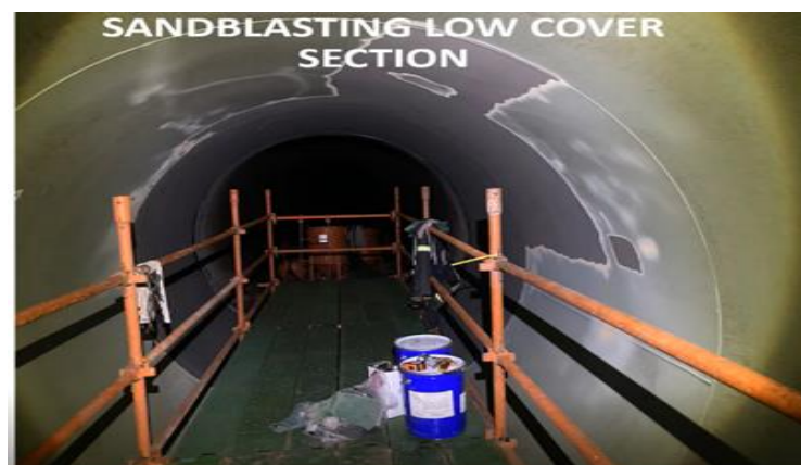
Figure 17 :Sandblasting low cover section
