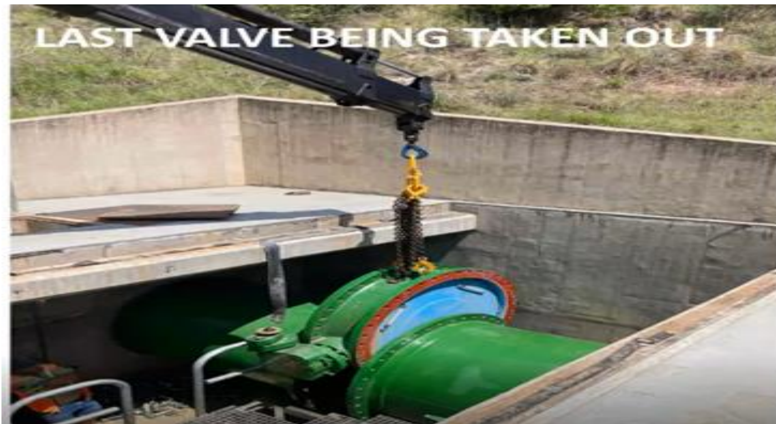
Figure 19: Last valve being taken out
